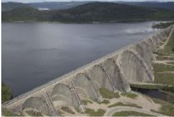
Hydro-Quebec Manic 5 Dam ( NHPR photo)
